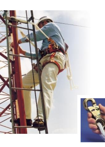
The cable is kept parallel to the structure along the entire length with cable restraints designed to keep the cable rigid, even in high winds. The ROHN-Loc Safety Harness and Safety Clamp securely lock onto the cable and the worker is secured to the structure.
